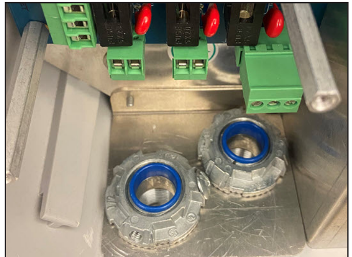
Figure 2: 1/2-inch conduit openings
