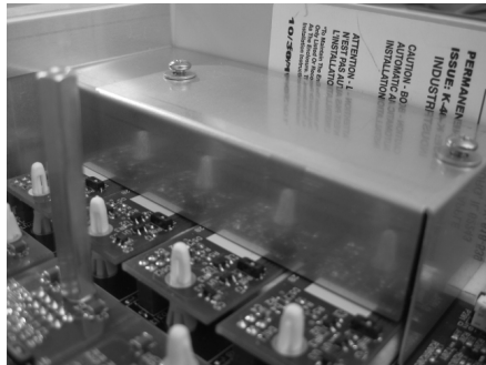
Figure 5 Installing the I.S. Cover
