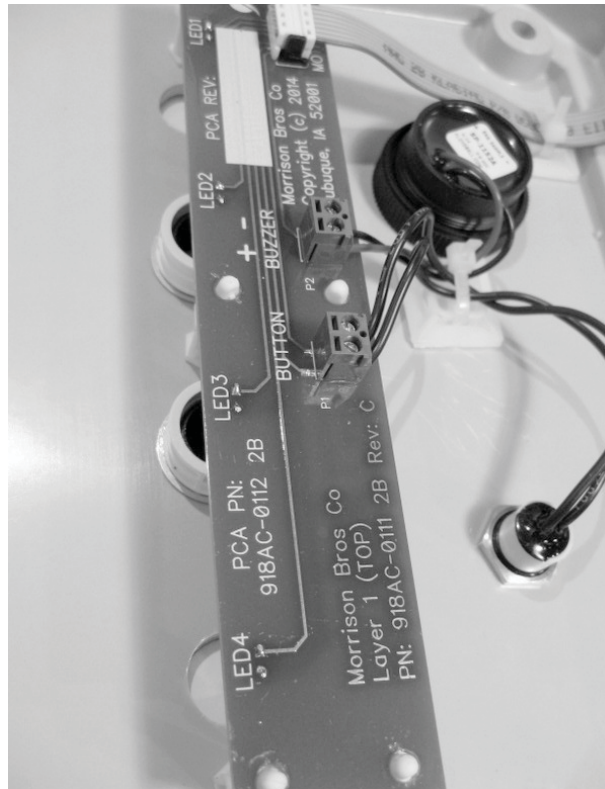
Figure 24 - Board is completely released and ready to be removed
